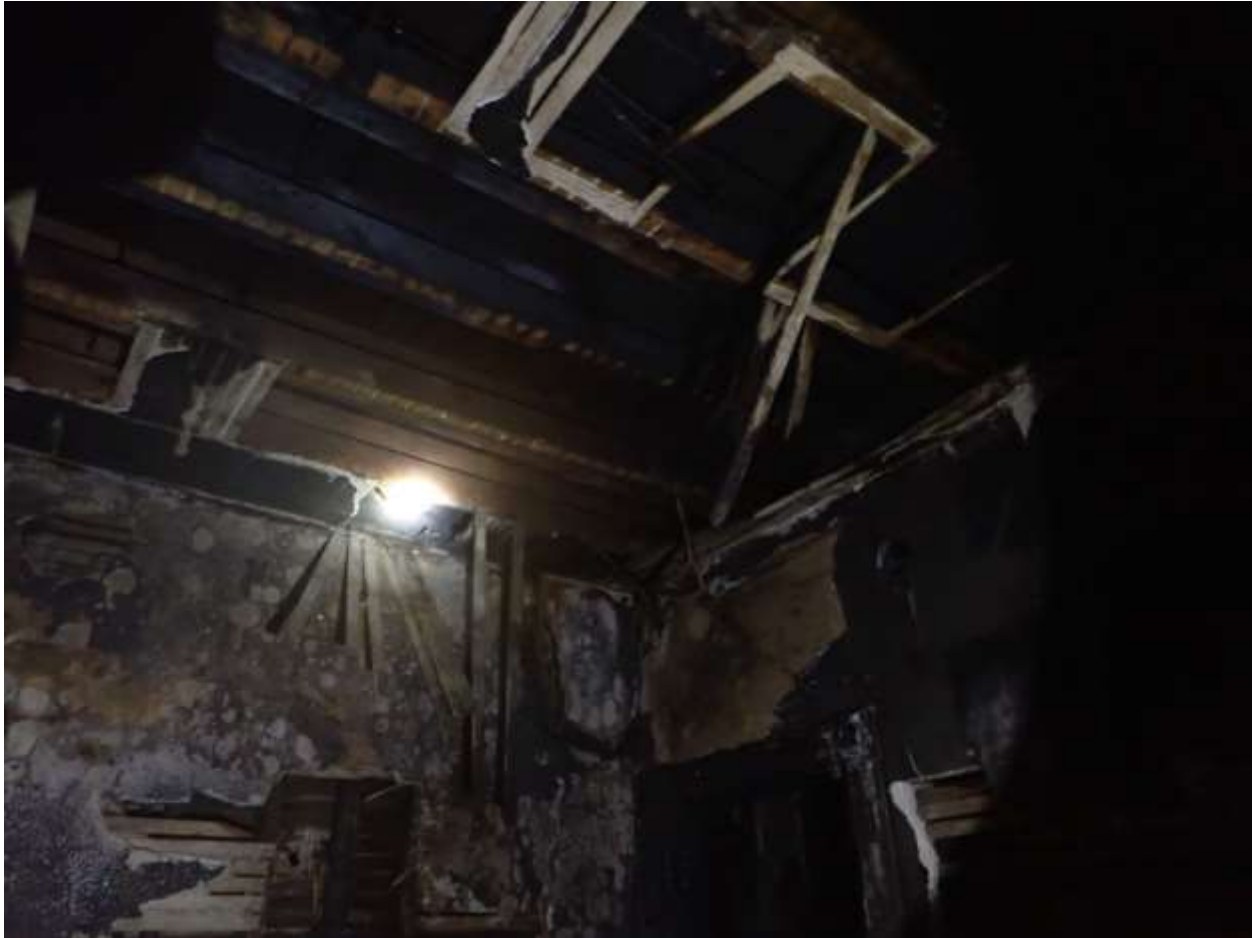
326 Charles Ave – Fire photos sent on 7/11/23
